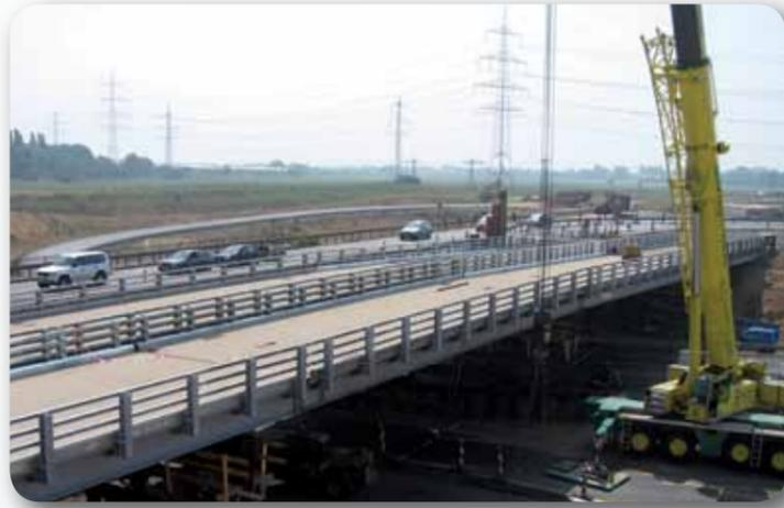
Janson's Plate Girder Bridge units (code JSB) are designed for temporary and permanent applications particularly in areas of heavy traffic conditions where single spans up to 40 meters for all general traffic are required.
