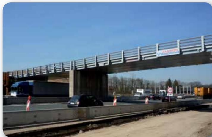
Janson's Beam Bridge units (code JSK) are designed for temporary and permanent applications wherever short span bridges up to 21 meter for all general traffic are required.
