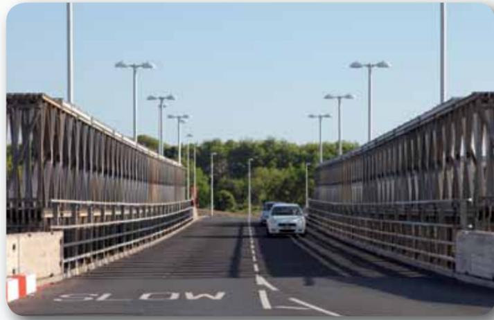
Janson's Panel Bridge system (code JPB) is designed for temporary and permanent applications wherever bridges with spans up to 400ft (122 meters) for all general traffic are required. The system is based on the original Bailey Bridge concept using trusses assembled from modular panels.
