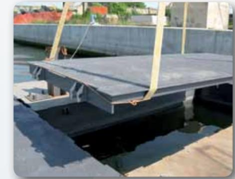
winches are available for the movement of platforms. Special infill deck elements can be used to increase stability and surface area reducing the number of pontoons required in a platform where a high floating capacity is not required.
