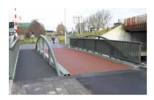
With its durable and low-maintenance properties, the JCB wins over bridges made of wood, steel and concrete. An actual maximum span of 40 meters can be realized. The width has no limitations, because the various elements can be connected to each other.
